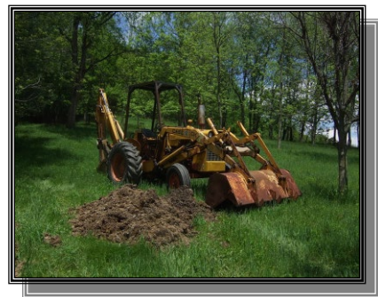
Photo 18 B frankenstoen (Flickr: backhoe)
